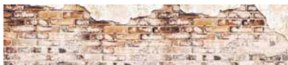
323 Ziegelwand 323 Brick wall
